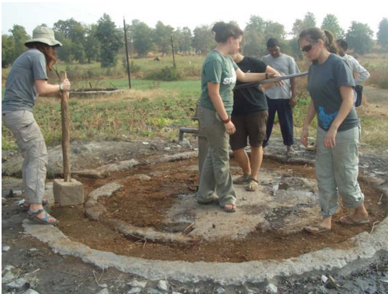
Re-cementing a water pump in Chilati, India.
